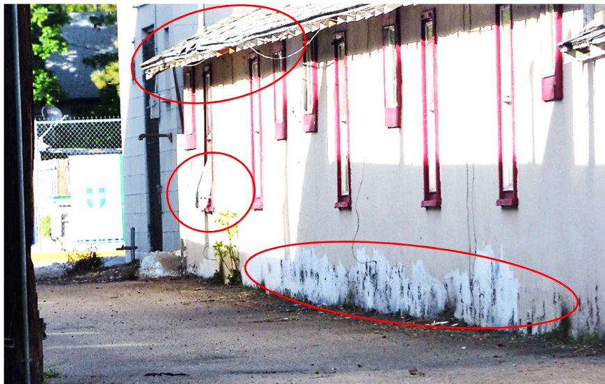
Deteriorating roof, walls/paint, fascia, windows
