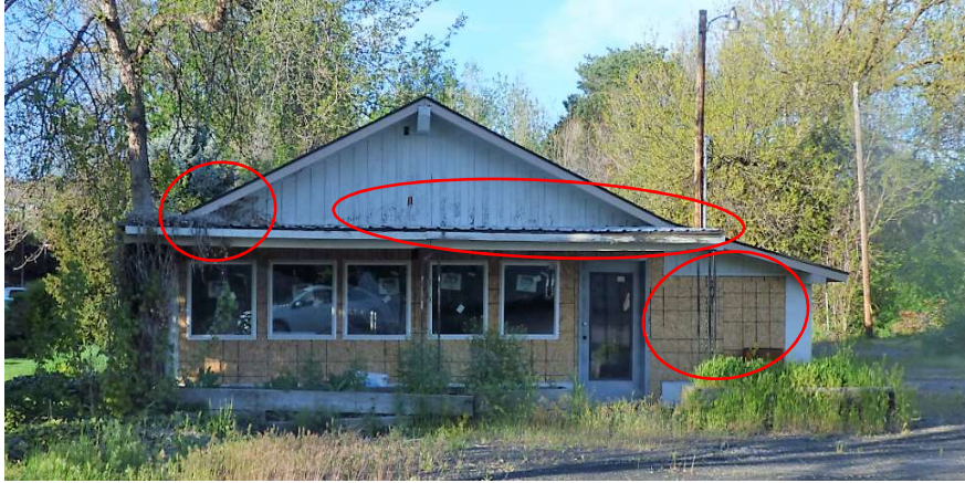
Deteriorating fascia/soffits, roof, walls, etc.
