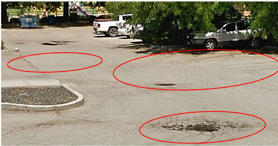
Deteriorating parking surface with faded/missing space markings
