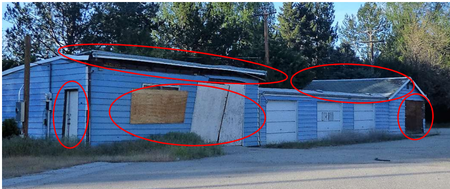
Deteriorating windows, fascia/soffits, roof, walls, etc.
