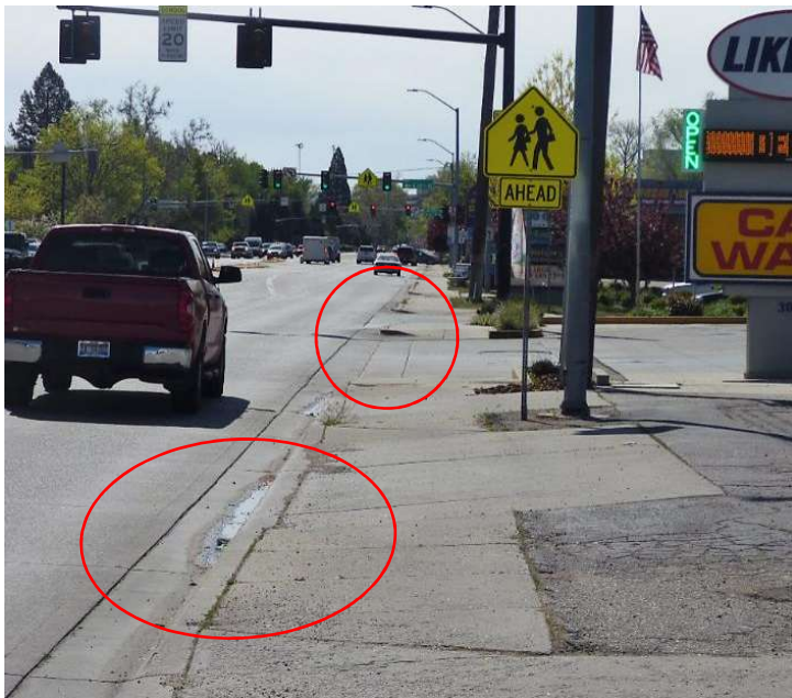
Sidewalk with multiple access points, loose gravel, deteriorated crosswalk striping, and little physical separation from heavy traffic
