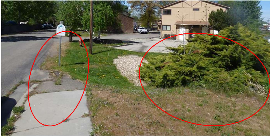
Cracked sidewalk, abrupt sidewalk end, deteriorating gutter, site/landscape maintenance
