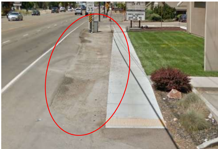
New sidewalk, but street margin deterioration and no curb/gutter
