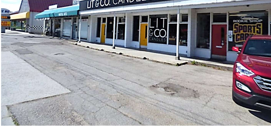
Deteriorating parking surface with faded/missing space markings
