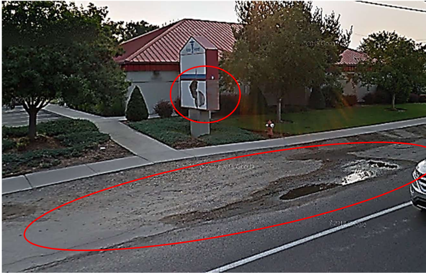
Sign damage, deteriorated street margin, drainage problems
