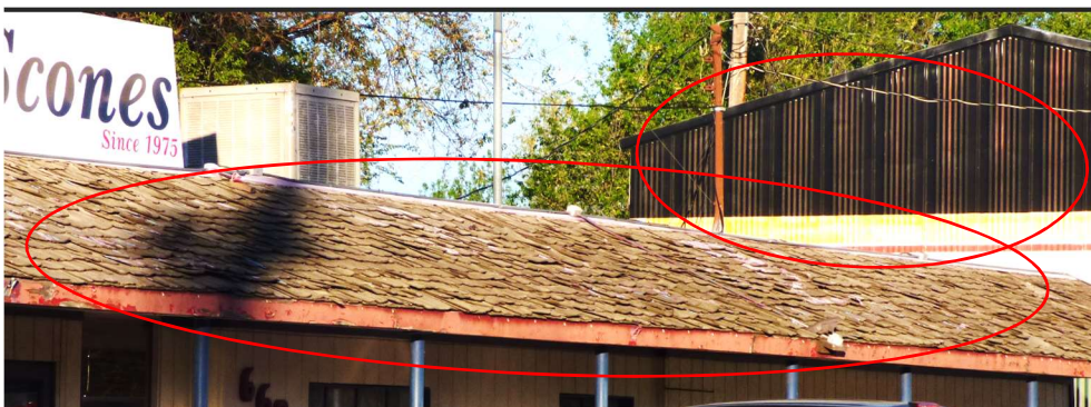
Deteriorating roof, fascia, paint; rusting wall (background metal structure)
